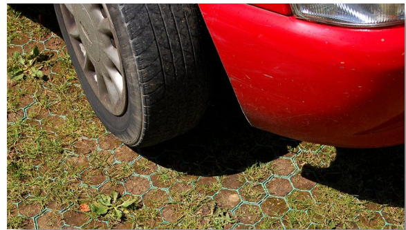
This driveway with permeable/porous covering helps reduce polluted runoff by allowing stormwater to soak into the ground.
