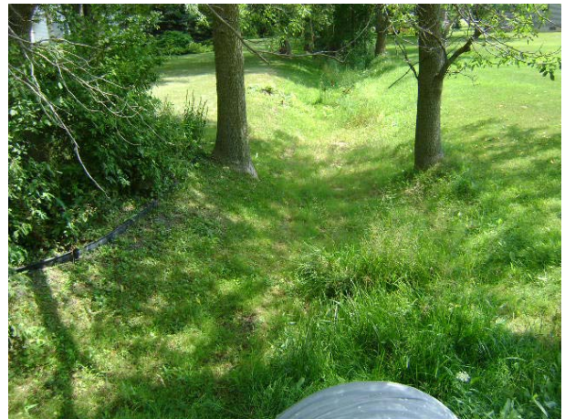
Harding Drain & VanVleet Rd.
