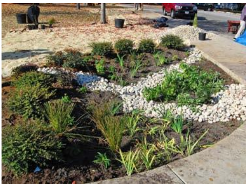
Bioretention areas, also called rain gardens, collect stormwater and filter out potentially harmful pollutants. (Photo: Chesapeake Bay Program)
