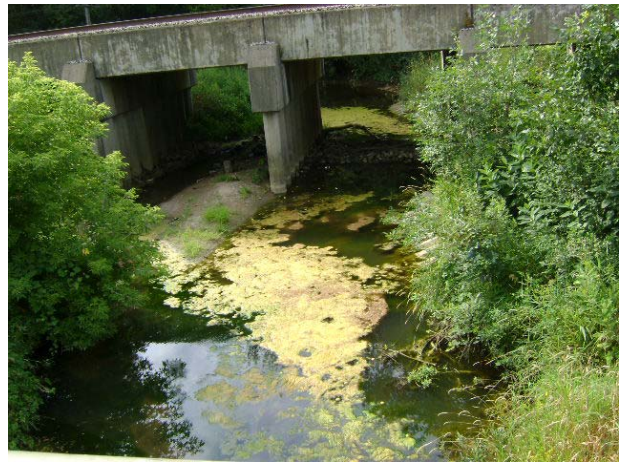
Jones Creek and Reid Road Crossing
